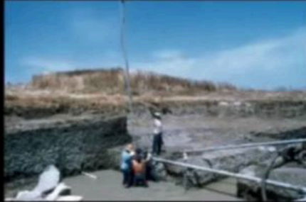
Installation of well point
